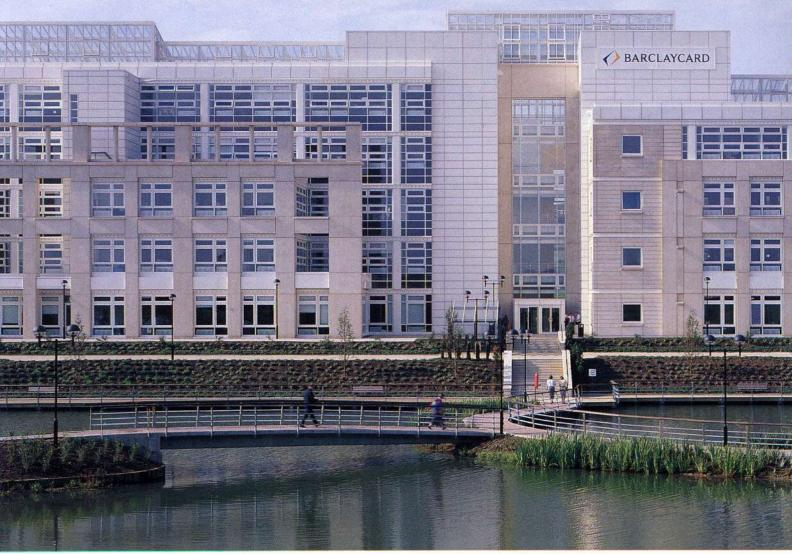
**Above** North facade. Water from the lake provides top-up cooling as required via chilled beams.
