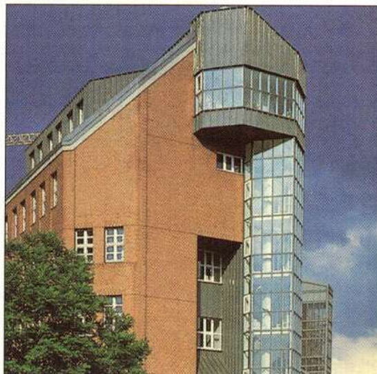
Part of the new Museum of Transport and Technology, Berlin, which is being built largely without PVC.
