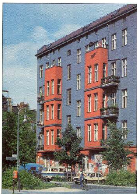
Social housing project for young people in Schöneberg, Berlin. The restored building is completely PVC-free.
